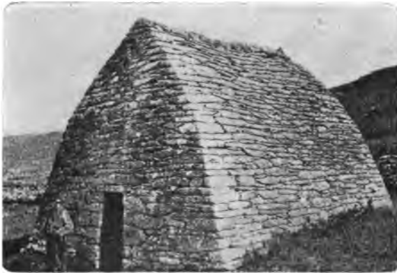
FIG. 21.—The Oratory of Gallerus, still standing in England. The shape of this house, in stone, is the same as that made by bending sapling trunks and tying the tops together.
